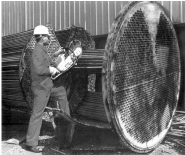
Figure 1: Abrasive disc cutting
