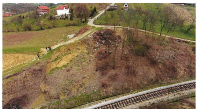
Fig. 16. Picture of landslide taken from UAS
