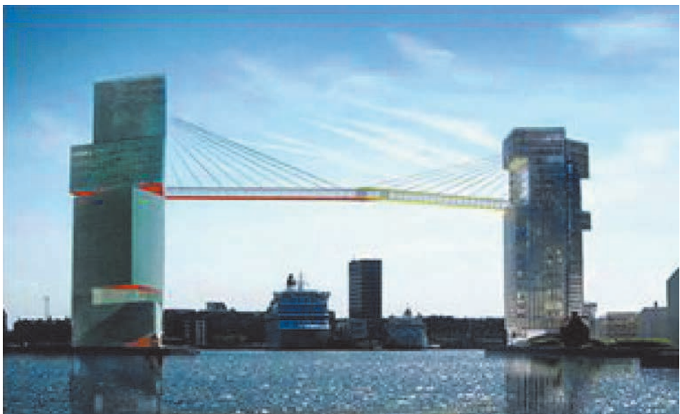
Fig. 14 – Stiphen Hools proposal for a inhabited bridge in Copenhagen (2008). The structure holds economic self keeping technology, wind turbines, photo volatile skyscraper casings. There are public spaces, offices, shops, terraces, various pedestrian communications, excavators, elevators and pathways. [22]
