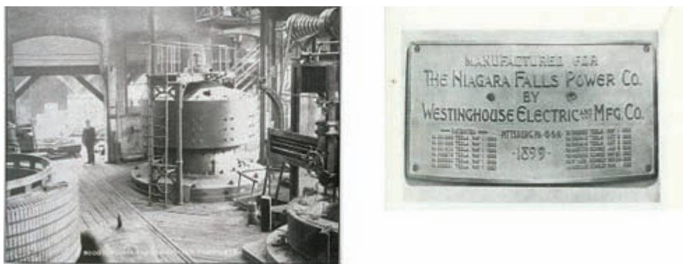
Figure 5. Interior of the turbine hall of Niagara Falls HPP and the name plate of Westinghouse Co. with the list of applied Tesla's patents
