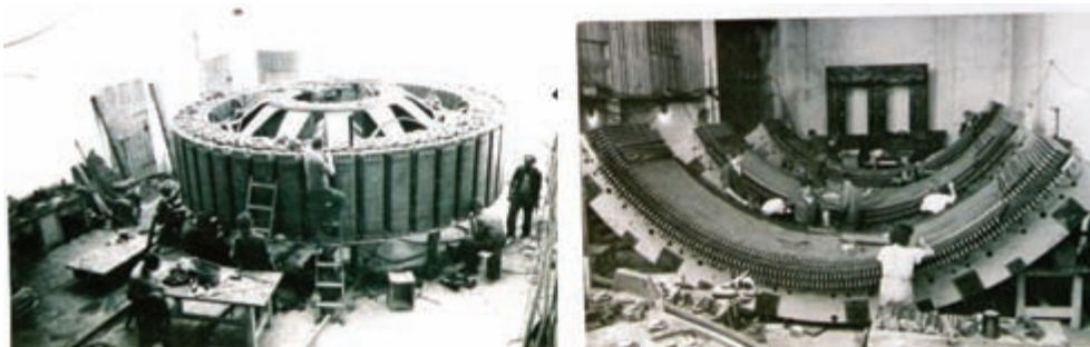
Figure 7. Manufacture of stator and rotor of 24 MVA, 10 kV, 125 r.p.m. synchronous generator for Mariborski otok HPP (1946)
