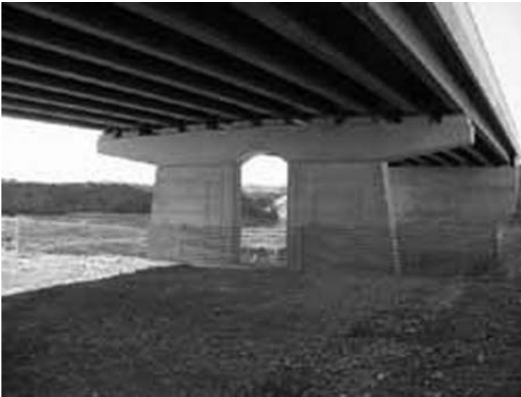
Figure 6: The view of Bourg-Les-Valence Bridge in France, the first European bridge to be constructed of ultra-high strength concrete
