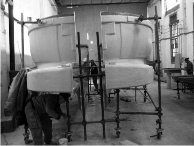
Figure 11: Completion of the moulds
