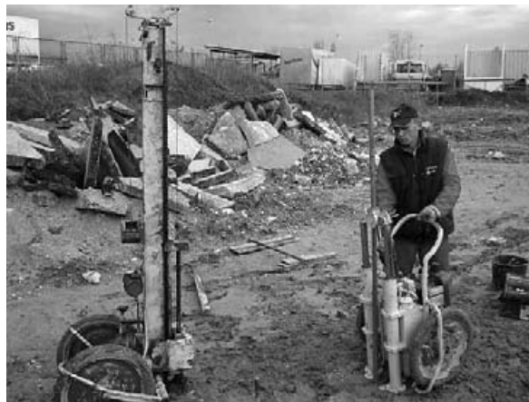
Figure 7: Soil improvement quality control by heavy impact probe
