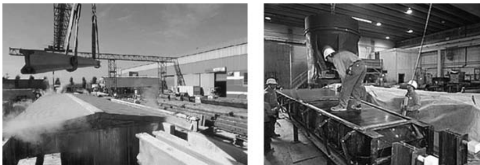
Figure 5: Production of girders made of ultra-high strength concrete
