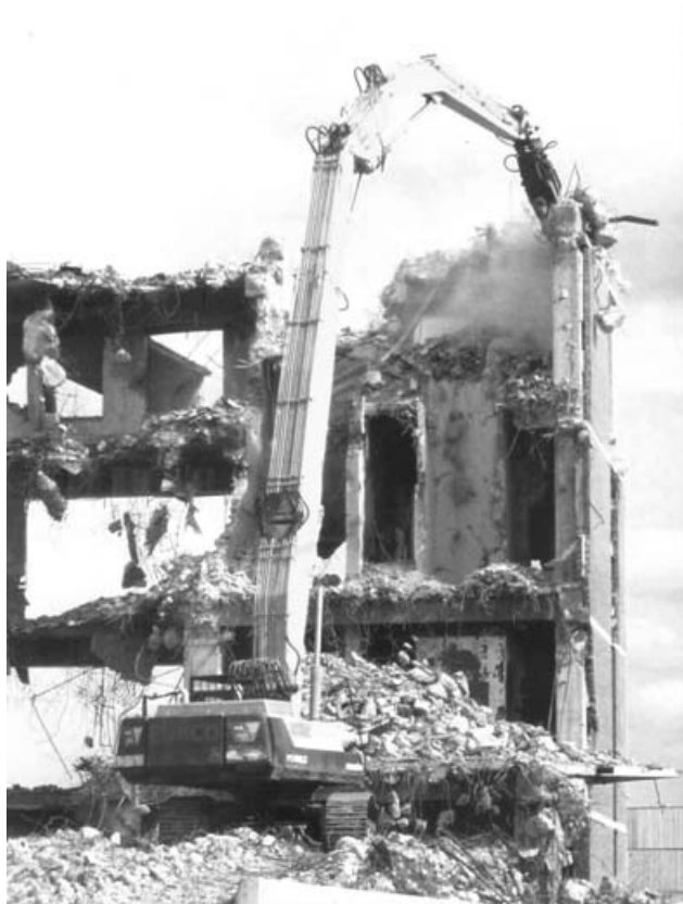
Figure 3: Crane-attached shear
