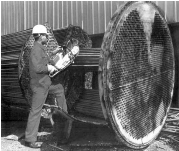
Figure 1: Abrasive disc cutting
